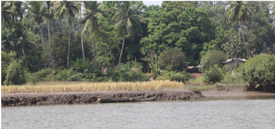
Figure 2.3: Landscape typical of the Great Scarcies river where the mangroves on the banks have been replaced by rice farming. Note the erosion of the unprotected banks. The dwellings are usually on higher grounds and populations have access to other type of wood thus they do not see the direct benefits of mangrove restoration, rather see it as competition with rice farming.
