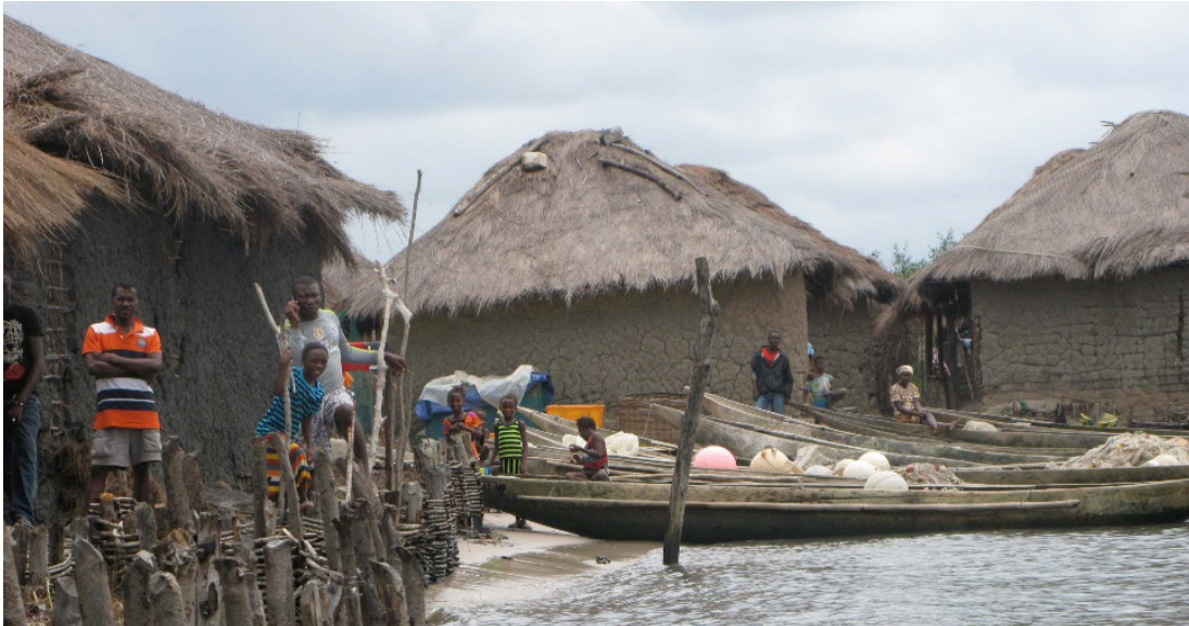
Figure 1.1: General view of the village of Njajeiam This view is typical of fishermen villages surveyed in this VA: dense build-up only few feet above the water level. Visible on the foreground are makeshift protections from the impacts of waves and storm surge. July 2016. Credit: S. Trzaska.
